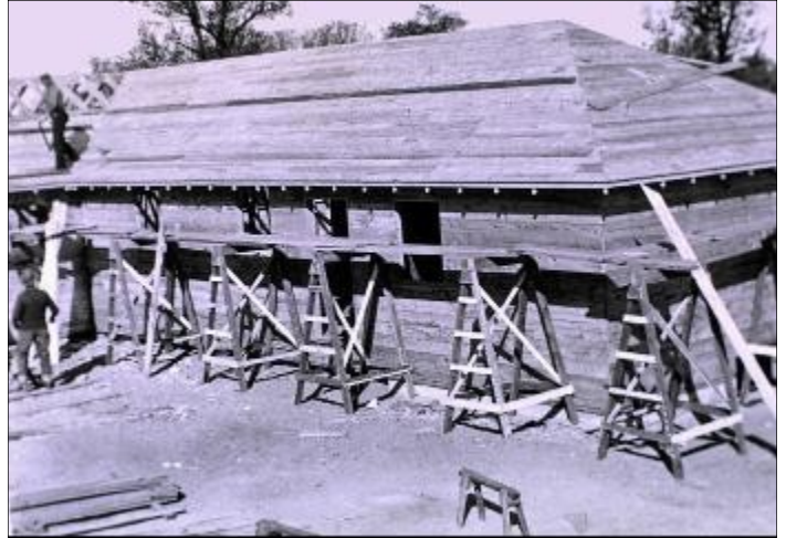
Mill Lake dining hall under construction in 1936
